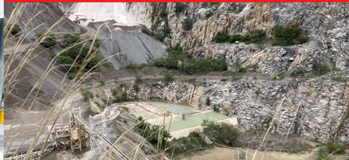
Tecolotlán Plant rainwater harvesting storage tanks.
