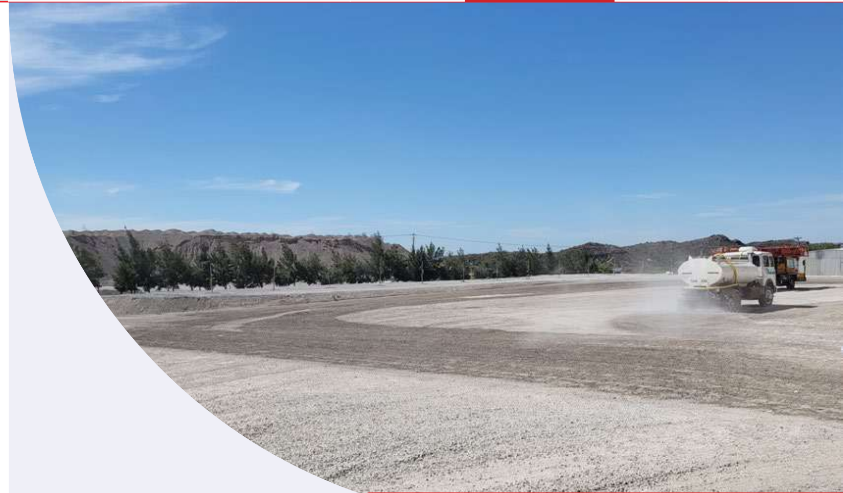
Treated wastewater is used to irrigate roads, Padre Bueno Plant
