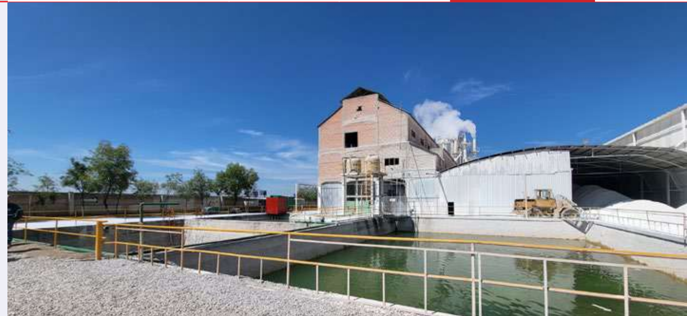
Water storage basins for rainwater harvesting at the Aguascalientes Plant.
