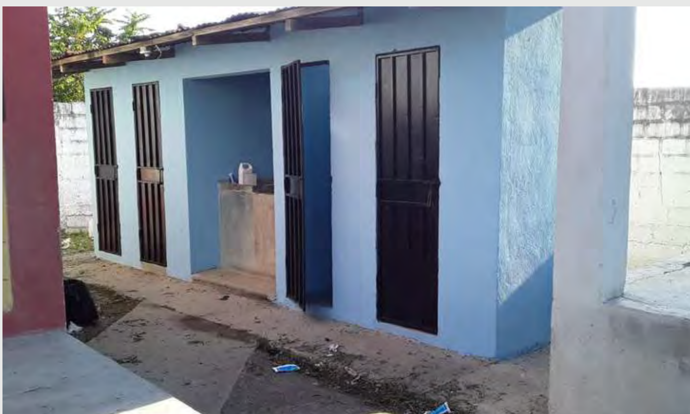
Remodeling of restrooms at Emilia Puerto School. INCAL Plant, Honduras.
